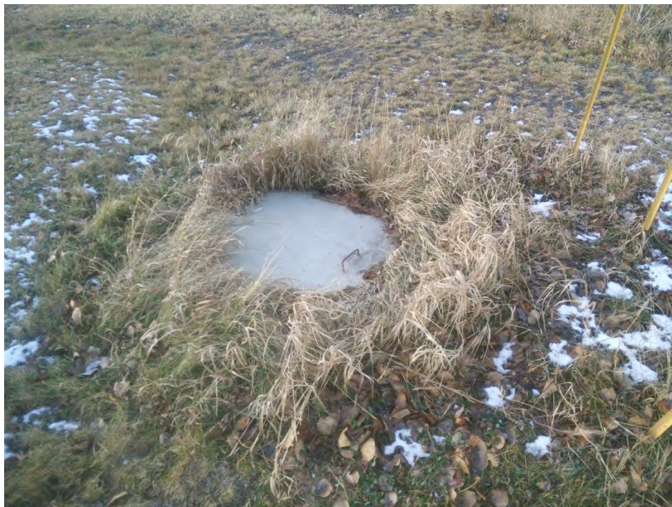
Photo 16 – View of the buried septic tank, located adjacent to the farm residence.
